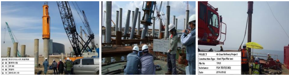
PDA Test for precast pile : Vertical & Raked pile
